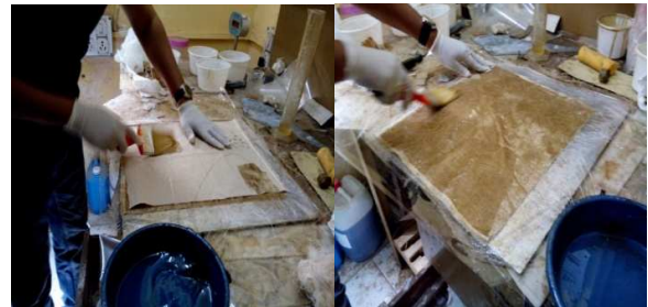
Fig 3.1: Applying epoxy polymer resin with help of brush layer by layer
